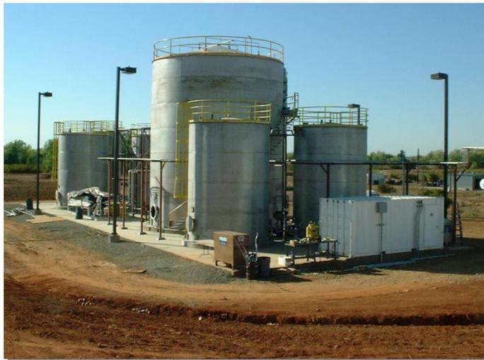
During Phase 2, the “baseline” wastewater in the feed equalization tank was supplemented with process wastewater containing a high level of TOC (i.e., greater than 10,000 mg/l) and salt (based on measurement of conductivity). The objectives of Phase 2 were to assess MBR performance in response to higher TOC and salt concentrations and to develop design and bioprocess control information.
