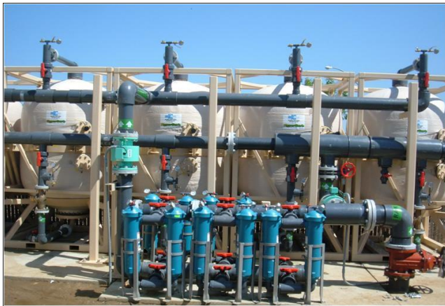
HyperSorb™ Uranium Removal System Ceres, California Water System
