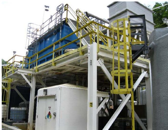
**Figure 4. Ballasted Sand Clarifier**
