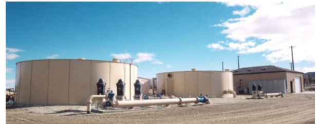
Envirogen's 2,500-GPM Nitrate Removal & Blending Facility
