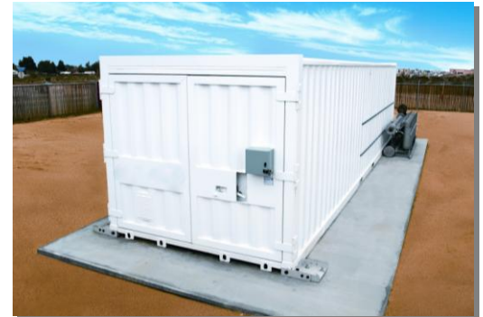
The first large arsenic removal system to be permitted in California was a 1,000-gpm system installed for the Victorville Water District by Envirogen.
