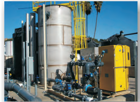
Nitrate Treatment FBR - San Diego, CA
