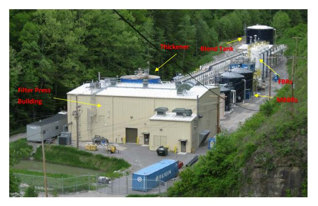
Figure 2. Overall Plant Layout – Selenium WTP
