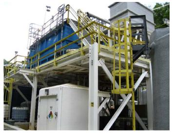
gravity settling systems that increase the terminal settling velocity of biological flocs, thereby minimizing system footprint. The clarifiers are used to remove TSS from the FBR effluent, which contains both excess (i.e., sloughed) biological solids and particulate selenium. The water is split evenly between two (2) units, each rated for 1,400 gpm (50% of maximum design flow). In each unit, the water flows through a series of chambers for coagulation, flocculation, maturation and settling.
