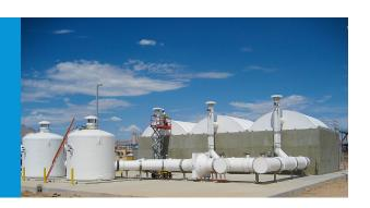
Envirogen Built-in-Place Biofilters are custom designed solutions for mid- to high-air flow VOC and odor control applications. These systems are employed in point source or centralized emissions control applications, for air flows ranging from 2,000 to well over 100,000 cfm. Installations are based on standardized system components and multibay designs to lower installed costs, increase flexibility of design and allow for expansion as plant needs change.
