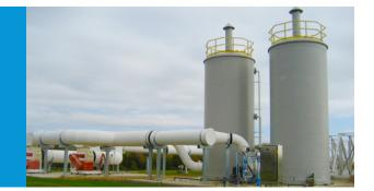
Envirogen Biotrickling Filters are vertically-oriented vapor-phase bioreactors filled with an inorganic media featuring 100% recirculation. The filters' unique design can address high concentration of H2<sub>s</sub> odors in areas where space is at a premium – offering a shorter retention time and treatment of higher air volumes than conventional biofilters. They can also treat high concentrations of VOCs and ammonia, and be chemically augmented when needed.
