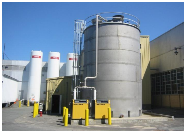
Bioreactor treating soft drink bottling plant wastewater
