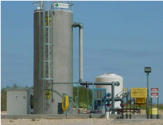
Envirogen Technologies, Inc.'s FBR Model EFB-7.5 system
